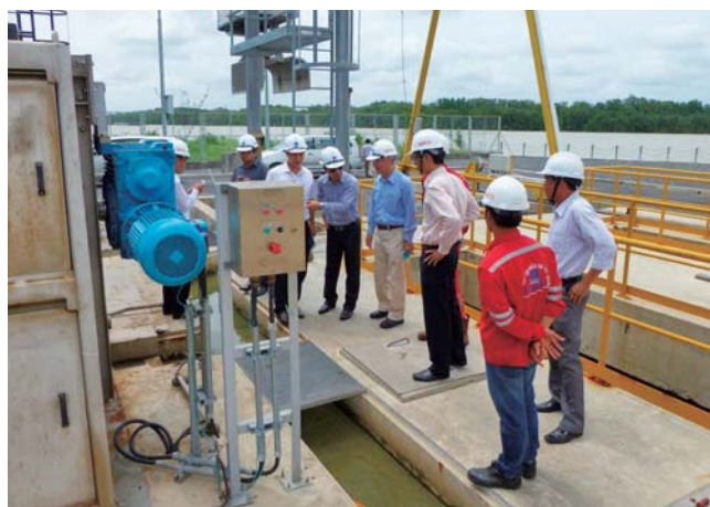
Onsite case study at Nhon Trach Power Plant
