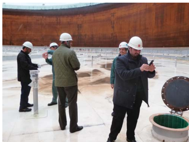
Tank maintenance site (Kiire Terminal)
