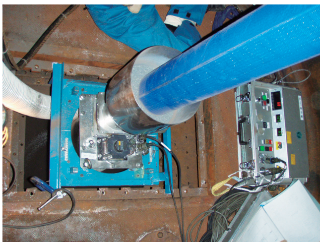
Catalyst dense loading (inside the reactor)
