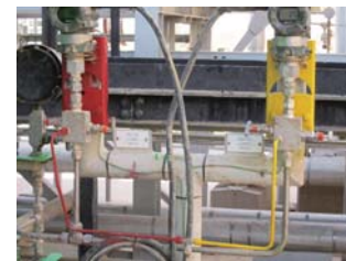
After improvement of the compressor area
