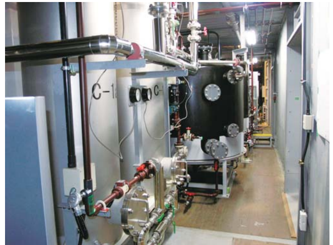
Wastewater treatment pilot plant
