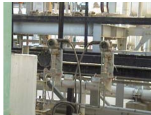
Before improvement of the compressor area
