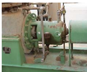
Before pump improvement
