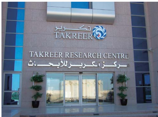
TRC building (3 stories): completed in April 2009 in the eastern suburbs of Abu Dhabi
