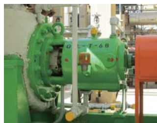
After pump improvement
