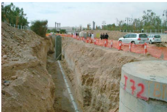
Site of sewage pipe installation work in Al Ain (pipes and manholes before being buried)
