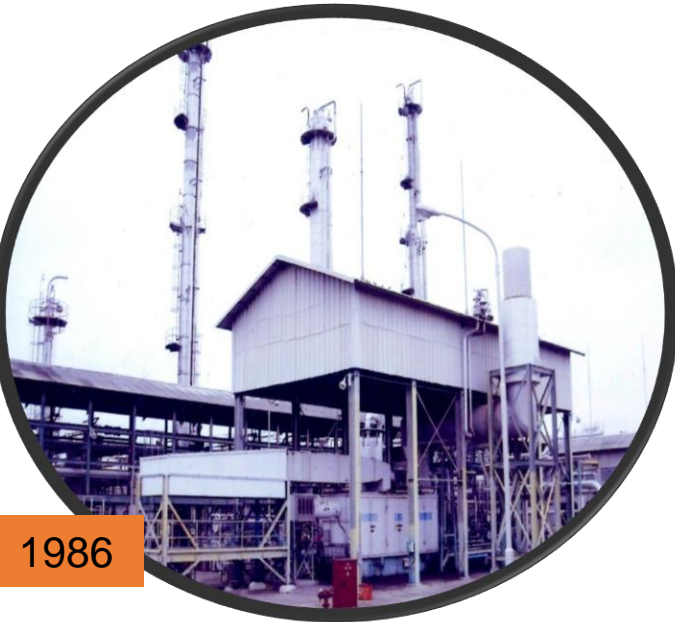
No(1) LPG Extraction Plant (Minbu)
