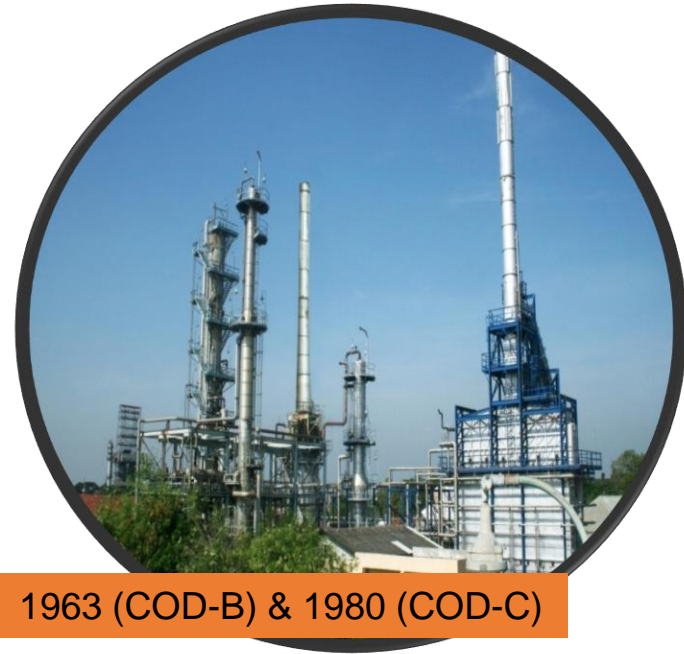
No(1) Refinery (Thanlyin)
