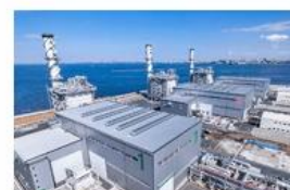
▲ Goi Thermal Power Plant
