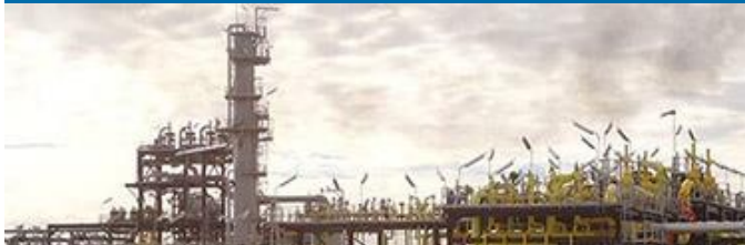
Gas Processing Plant for Sonatrach, Algeria
