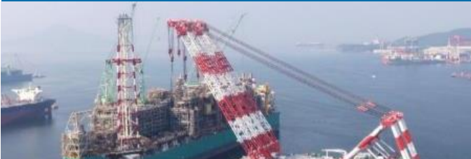
FLNG Plant for PETRONAS, Off the coast of Malaysia
