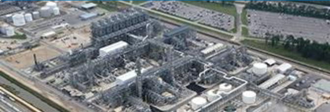
Ethylene Plant for Chevron Phillips Chemical, US
