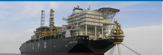
LPG FPSO Plant for IHI, Angola
