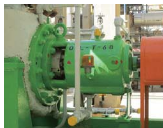
After pump improvement
