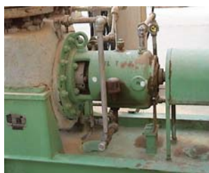
Before pump improvement
