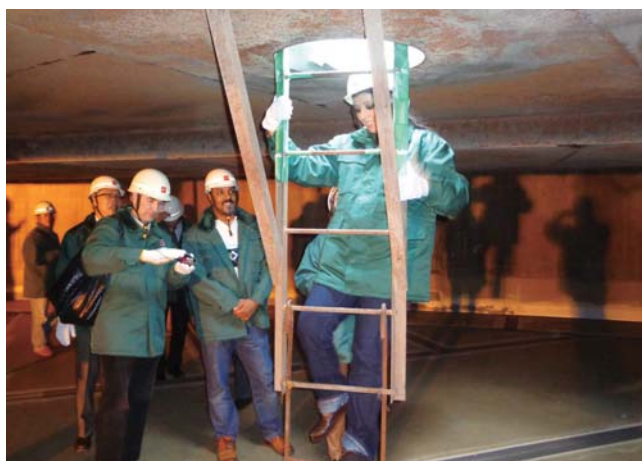
Inspection of a 100,000kL crude oil tank that is open for overhaul
