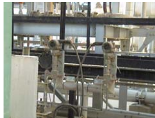
Before improvement of the compressor area
