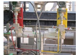
After improvement of the compressor area
