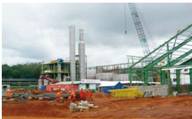
Construction site of the bioethanol plant
